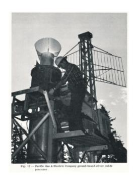
A PG&E ground-based silver iodide generator Image source: the Pacific Gas and Electric Company
